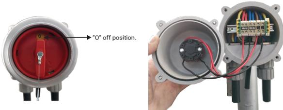
1. Remove the switch assembly by loosening the screws on the switch housing.
